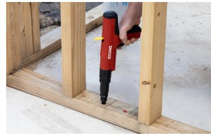
(f) fixing of timber frame to slab
