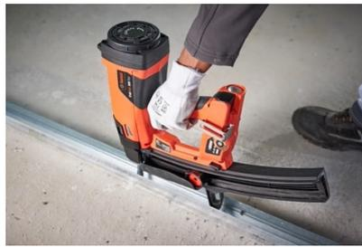
(e) fixing of steel frame to slab
