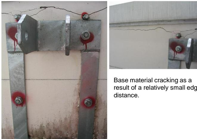
Base material cracking as a result of a relatively small edge distance.
