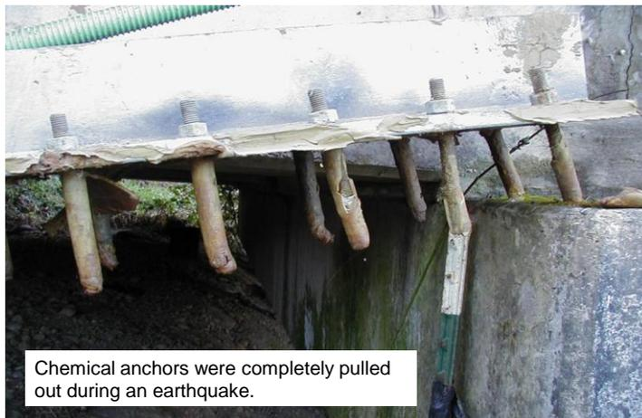
Chemical anchors were completely pulled out during an earthquake.
