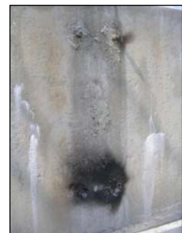
Torch cut anchors.
